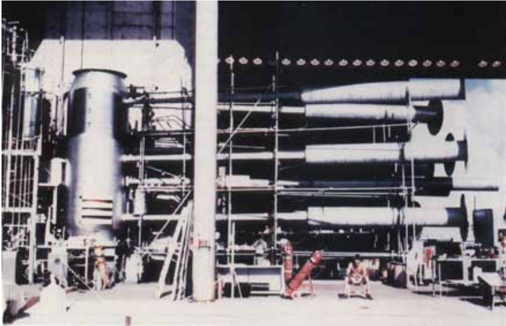
The prototype H-bomb, “Mike,” at left, 1952. The horizontal tubes will carry its light to special cameras two miles away for later analysis.
